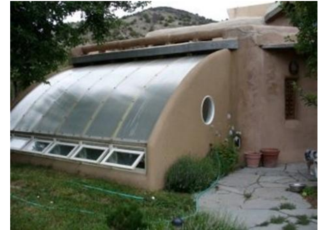
Figure 91 Example of sunken three-sided, closed greenhouse. Electronic reference: https://dekoriko.ru/
