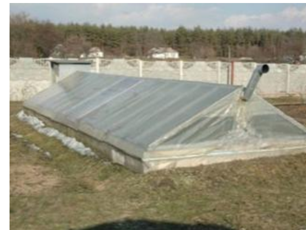
Figure 89 Example of sunken greenhouse. Electronic reference: https://dekoriko.ru/
