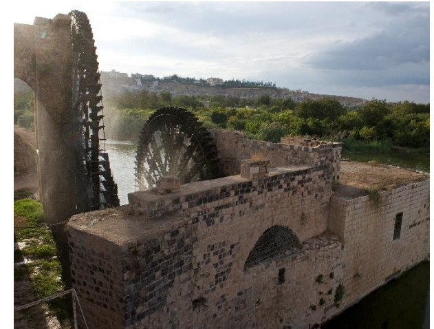
Figure 72 Aqueduct of Hama, Syria XIII century.
