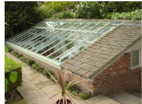
Figure 92 Example of sunken three-sided, closed greenhouse. Electronic reference: https://dekoriko.ru/
