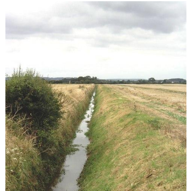
Figure 68 Drainage channel. © Wikimedia/ David Kemp https://commons.wikimedia.org/wiki/File:Drainage_channel_-_geograph.org.uk_-_530359.jpg
