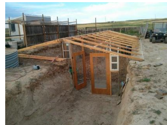
Figure 90 Example of sunken three-sided, closed greenhouse. Electronic reference: https://dekoriko.ru/
